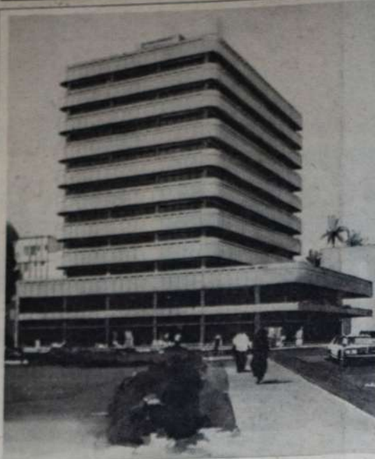
THE MOMBASA PLAZA, Aga Khan Road.
