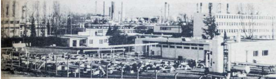
GAS: The recent find of natural gas in huge amount and concentration of space should lead France out of its energy crisis. Underneath the village Lacq, in the south-western French province of Aquitania, a field of natural gas of more than 200,000 million cubic metres has been discovered quite by accident. However, geologists believe that further boring down
