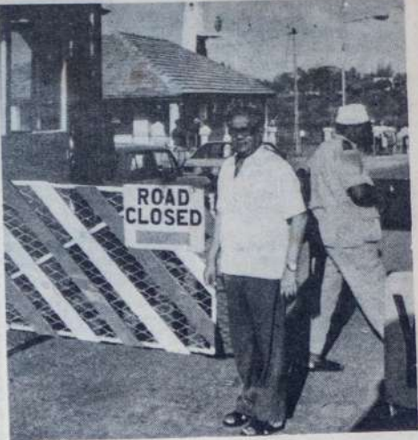
MR AMRITLAL SHAH is on the old Nyali Bridge. PHOTO: NATIONAL
