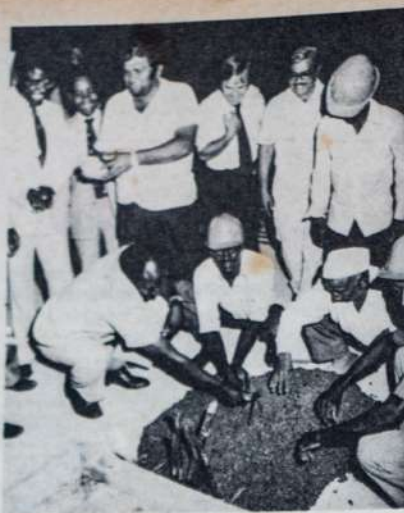
VICE PRESIDENT and Minister for Finance Mr. Mwai Kibaki is pictured while performing the 'topping off' ceremony on the eighth floor of the new Mombasa Plaza building, owned by the Kenya Re-insurance Corporation. He is flanked by Corporation executives and contractor staff.
