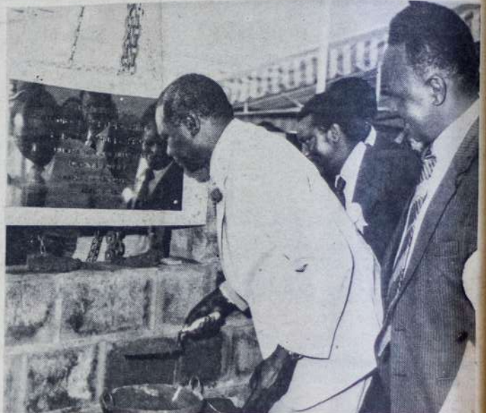
PRESIDENT MOI lays the foundation stone for the Kisumu Breweries complex.
