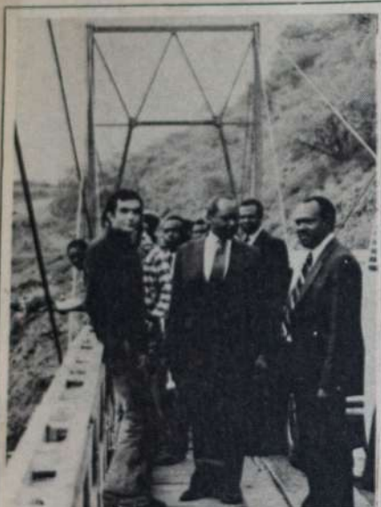
INSPECTION TOUR: President Moi looks over a new bridge under construction at Margat in Baringo District.
