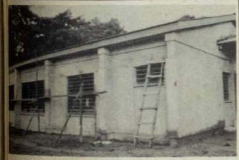
A Section of the newly completed Baby Wing at Mji Wa Salama.
