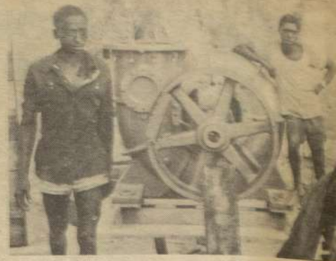
THE HUGE Kirloskar pump is seen during installation at Kurawa.
