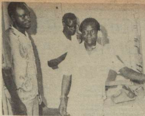
CHANGAMWE EXCHANGE - A two thousand line modern telephone exchange that will ease congestion at Moi International Airport Mombasa and the surrounding areas, has been commissioned by Mr. Michael Kilili, Head of K.P. and T. Corporation's Telecommunications Services, who is seen trying on headphones during the commissioning ceremony. Behind him is the K.P. and T. Corporation's D Coast Divisional Manager, Mr. Charles Muga. Looking on (left) is Mr. R.W. Sitati, Chief Major Works K.P. and T. Corporation.
