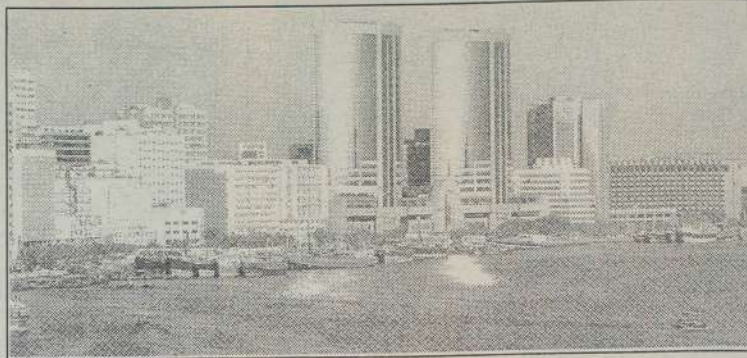
ULTRA-MODERN skyline of busy down town Dubai - Building activity is very noticeable as it is taking place virtually everywhere, mainly villas and flats.
