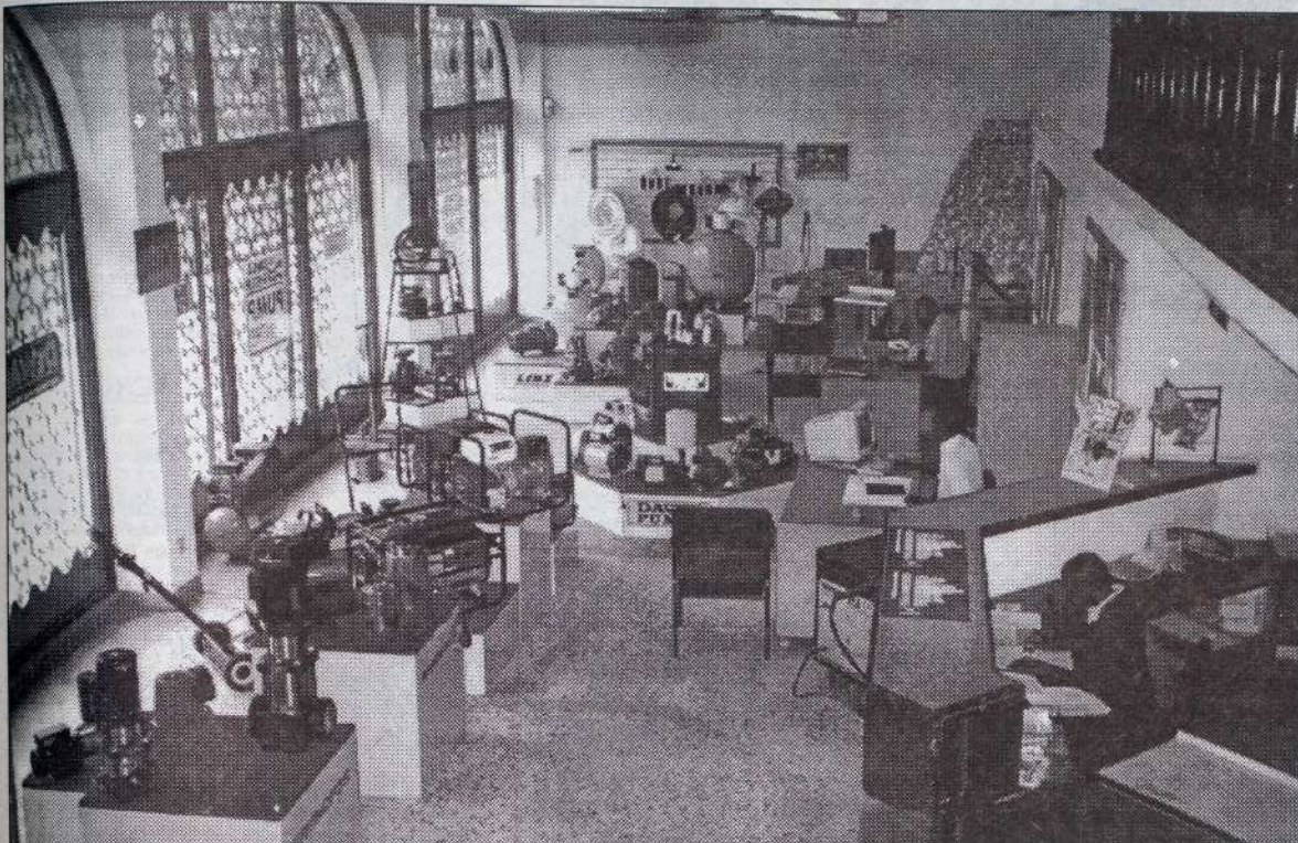
SMART SHOW ROOM in Butech's fully air-conditioned Jomo Kenyatta Avenue Head Office complex where salesman can demonstrate the latest equipment from such world famous names as Grundfos, Davey, Linz, Osaka, Flygt and Ajax pumps.
