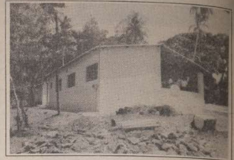
A MAJOR CONTRIBUTION to 'Health For All By The Year 2000 A.D.' for people in the Kariji Circuit of Ribe, Kilifi District, is this new Health Clinic which was recently completed by contractors working with plans and funds provided by the Mombasa Round Table No. 25. It is hoped that support staff duties will be provided by local people.
