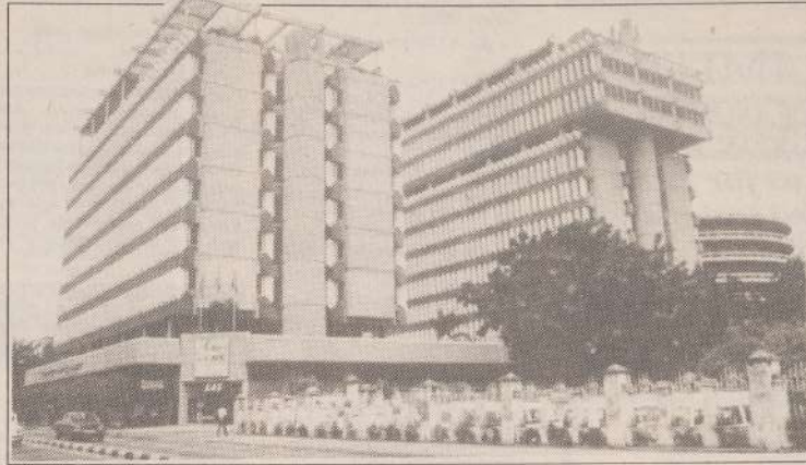
ONCE PRIDE OF MOMBASA the multi-storey Ambalal House is getting some much-needed improvement.
