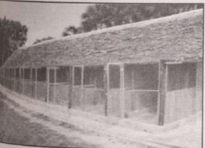
Above is the up coming Bamburi Cement Kennels which will accommodate over 100 dogs for Nyal and own area assignments.
