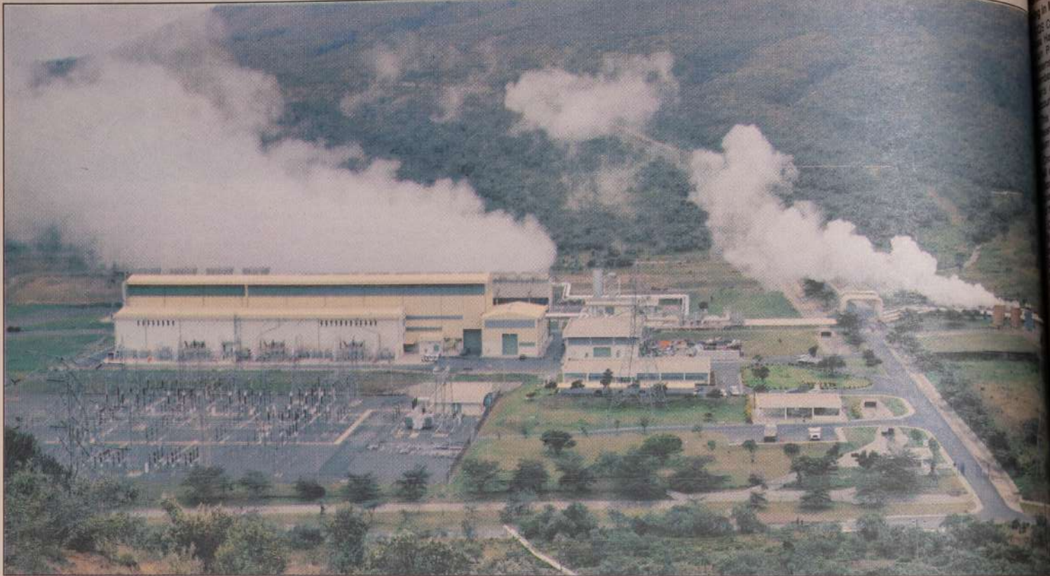
NAIROBI (Xinhua) — The Olkaria geothermal power plant is seen in Rift Valley Province of Kenya, on August 29, 2010. Seventy percent of the drilling work to create new geothermal steam wells in Olkaria geothermal power plant has been done. The new wells are expected to produce 280 megawatts of electricity within the next two years. About 33 steam wells have been drilled in Kenya since the exploitation of geothermal energy began in 1981. Kenya has the potential geothermal of 7,000 megawatts. XINHUA PHOTO - ZHAO YING
