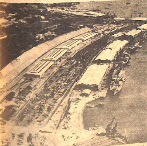
* DEEP Water berths and their accompanying transit sheds and rail yards line the harbour front. PHOTO: KENYA PORTS AUTHORITY
