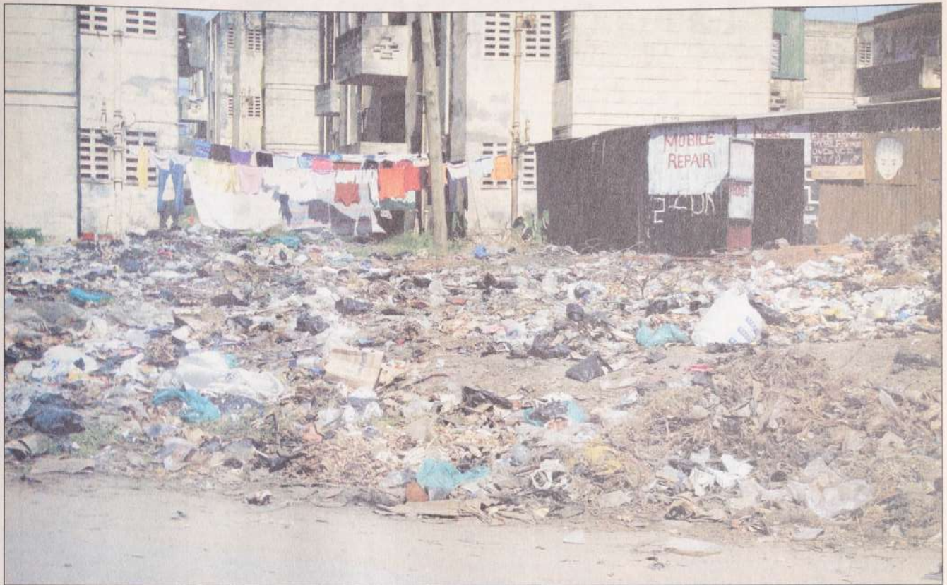
SLUM AREA NEEDS A 'CLEAN UP' - This is the shocking state of squalor with which South Coast residents at Likoni are only too familiar. The buildings are in an obvious state of disrepair and the scenic gardens have been turned into a huge and unseemly rubbish tip. Tourist being ferried to the plush South Coast holiday resorts frequently comment on this unsightly and festering eye sore, which lies adjacent to the main Mombasa Diani highway. It is hoped that Mombasa civic authorities will eventually get around to clearing up this mess?
