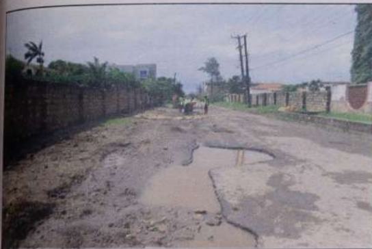
Waterlogged and deeply eroded condition of roads in Nyali residential area, where Kenya Urban Roads Authority workers are now sealing the potholes.
