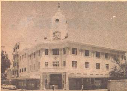
LANDMARK — The Swaminarayan Temple, near the Mombasa Rail way station has been completed redecored with Sadolins paints.
