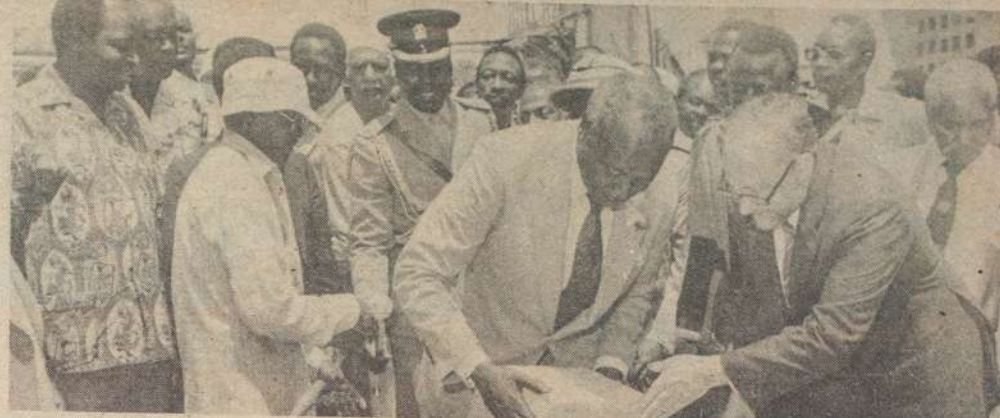
PRESIDENT Daniel Arap Moi is seen officially laying the Foundation Stone at the new Shs. 40 million Sheikh Khalifa Bin Zayed Secondary and Technical School now nearing completion at Bamburi, near Mombasa, on the Kenya North-Coast. Looking on are
