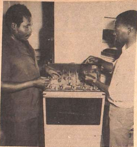
MR. T. KASSIM (right), the Car and General Manager in Malindi, is pictured discussing the repair of a gas stove in the firm's newly constructed workshop with Mr. James Adongo, an appliances technician. The workshop and a tyre store have been constructed to cope with Car and General's increase volume of business in Malindi.
