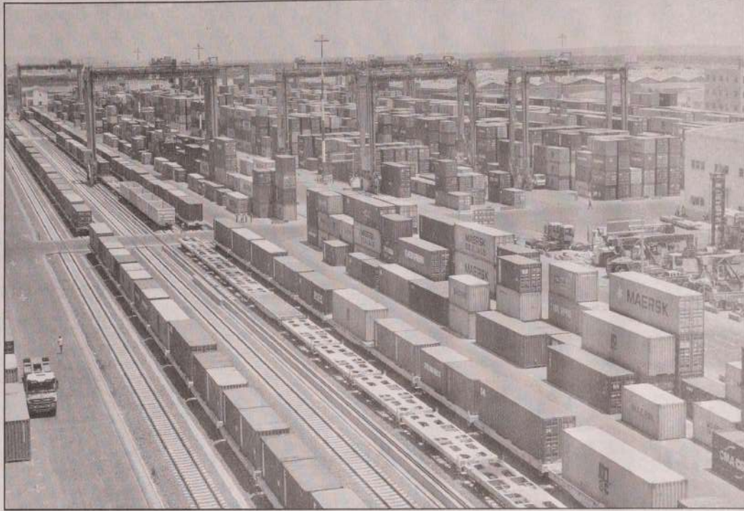
NAIROBI (Xinhua) -- Photo taken on Oct. 29, 2018 shows an overview of Inland Container Depot in Nairobi, capital of Kenya. The yard has a capacity of 14,000 Twenty Foot Equivalent Units (TEUs) and currently is holding 10,500 TEUs. XINHUA PHOTO - ALLAN MUTISO
