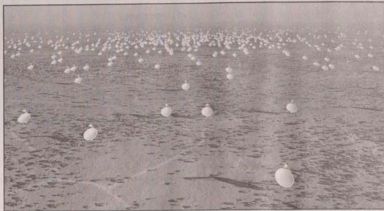
Artist's impression of the 5km diameter central core of Square Kilometre Array (SKA) antennas.
