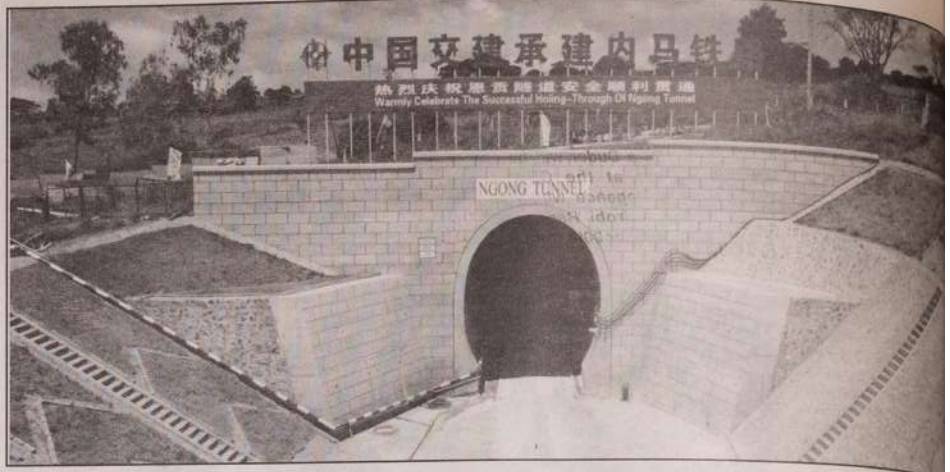
NAIROBI (Xinhua) -- Entrance of the Ngong tunnel [left] of the Standard Gauge Railway (SGR) in Nairobi. China Communications Construction Company (CCCC) has drilled longest railway tunnel in East Africa, the company said Monday. The tunnel is part of phase 2A of the Standard Gauge Railway that runs from Nairobi to Naivasha town. XINHUA PHOTO - WANG TESHU
