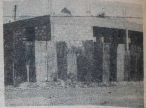
VIEW of the partially completed Tahdhib Muslim School.
