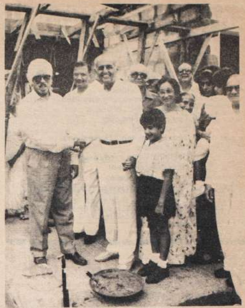
AFTER laying the foundation stone for the new Intensive Care Project at Pandya Memorial Hospital Mr Yusuf Mamujee of Mamujee Brothers Limited was thanked by the chairman of the Pandya Memorial Hospital's Board of Management Dalip S. Obhrai. He expressed gratitude to the Mamujee family for having made the largest single donation of Shs one million to this project. Mrs Y. Mamujee is seen second right.
